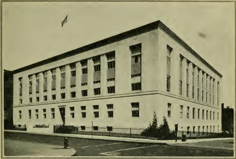
GENERAL VIEW—Showing the results obtained by the architect in using a modern classic design to produce a building of striking simplicity and beauty. In relief on each of the spandrels between the upper rows of windows are intertwined a gear and a governor, suggestive of the Company's business.
